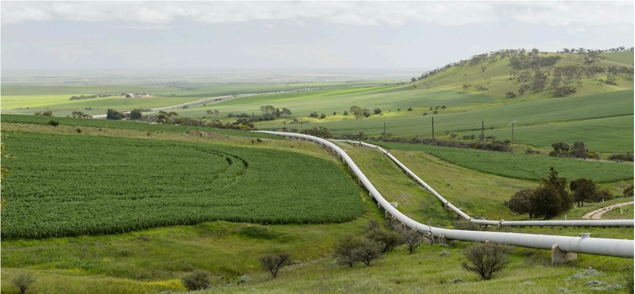
Morgan-Whyalla Pipeline, South Australia.
